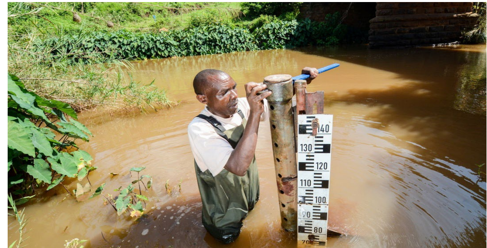
Figure 7 Colleagues at the Kenyan Water Resource Management Authority (WRMA) installing river gauge board holders in Tana river © CIAT/Georgina Smith
